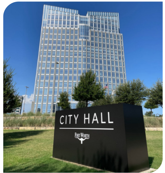
Fort Worth leverages the near real-time data to track continuous water use and alert customers of any potential issue.
