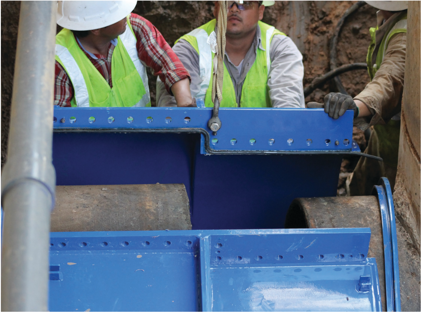
On this project, Smith-Blair was called in to resolve a connection that failed due to pipeline settlement. The split offset coupling pictured here permanently connected and sealed the pipeline without removing the existing pipeline or fittings.
