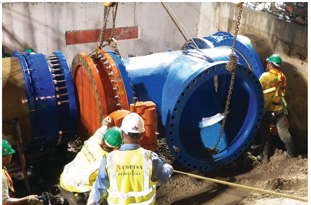
On this project, Smith-Blair was called in to resolve a connection that failed due to pipeline settlement. The split offset coupling pictured here permanently connected and sealed the pipeline without removing the existing pipeline or fittings.
