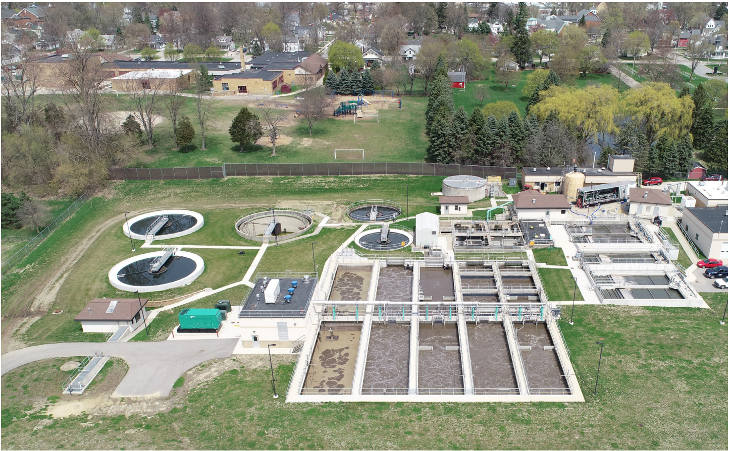
An aerial view of the Zeeland Clean Water Plant.
