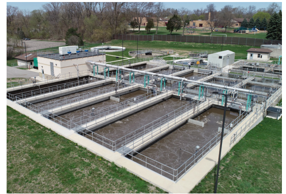
Primary sedimentation tanks which allow heavy debris to float to the bottom to treat wastewater.
