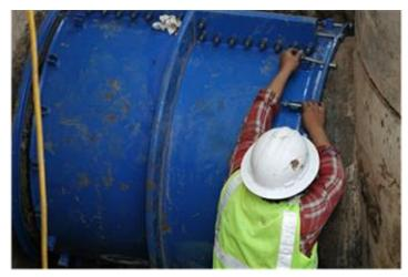
The photo shows the contractor installing the end rings to complete the process. Smith-Blair manufactured the sleeve for a perfect fit (including length) while allowing enough room to bolt the split sleeve together with ease in the limited space.
