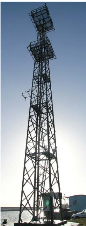
Fig. 6A: Wind and Weather sensors installed 15m above ground level
