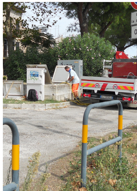
The Squero wastewater pumping station
