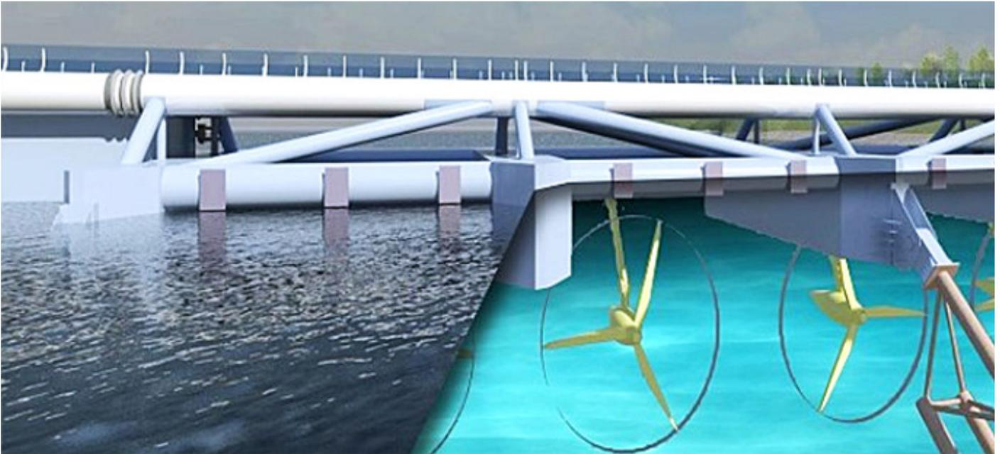
Conceptual design of the 800m floating bridge crossing the Lantuka Strait and connecting the islands of Flores and Andonara. The bridge would include a tidal energy power plant with a capacity of 18 to 23 MW.
