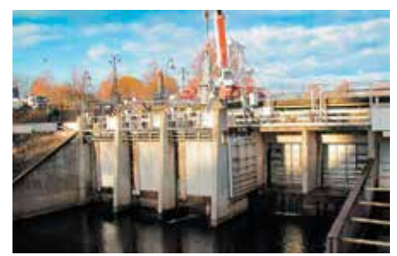
Potable Water Pumps & Drinking Water Treatment Systems
