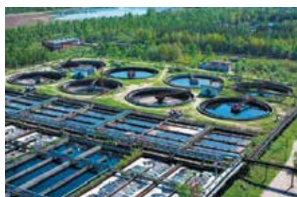
Municipal Wastewater Pumping & Treatment
