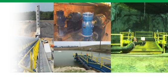
At the mixing chamber, the mine water was diluted by fresh water and then pumped by an additional vertical turbine pump to a fine refuse impoundment site for filtering impurities, to a settlement pond for storage and finally to the preparation plant for washing coal. At the settlement pond, Flygt submersible pumps floating on Xylem custom barges - designed to keep the pumps at the proper submerged level - ensured that the preparation plant would receive clean washing water.
