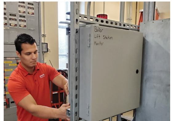
NEMA 4X control panel being installed on Rice University campus.
