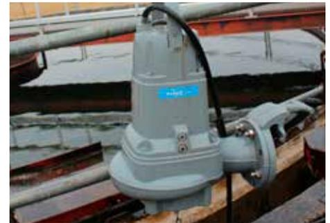
Concertor® pump being removed after 1 month of operation for inspection.
