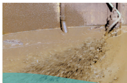
Liquid manure pumps
