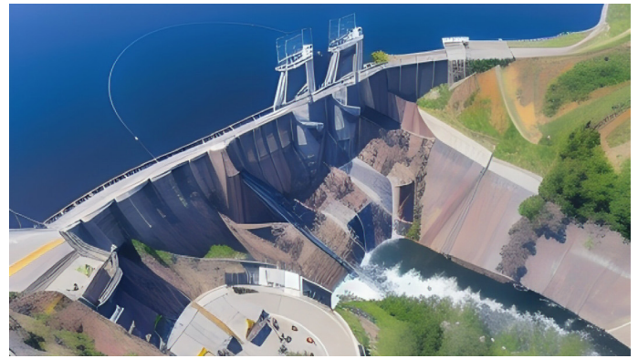
The John Hart Dam in British Columbia, Canada, was recently upgraded to a run-of-river hydropower system.
