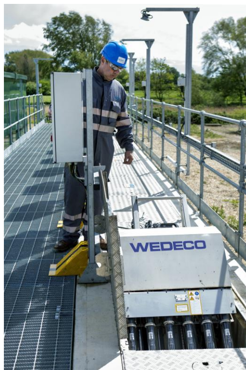
Integral automatic lifting provides comfortable access to all UV module components
