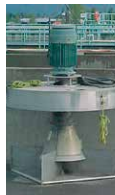
Old surface aerator removed from digester no. 1.
