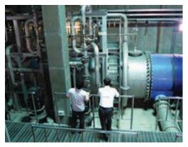
Two ozone injection lines with a flow rate of 17,000  $\ensuremath{\mathsf{m}}^3/h$  each.
