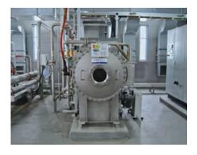
Three WEDECO PDO 1000 ozone generators are producing up to 51 kg of ozone per hour from liquid oxygen.
