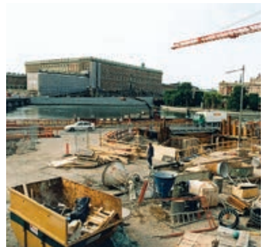
The building site with Stockholm's Royal Castle in the background.
