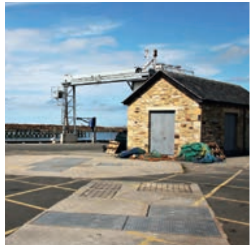
NWL’s maintenance project involved seven pumping stations.
