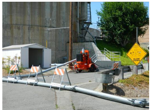
NC150 Dri-Prime pumping into City-owned Godwin Bauer 8" Quick-Disconnect pipe.
