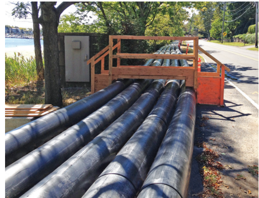
The eight-week bypass system employed 11,000 ft of HDPE pipe.
