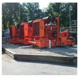
Bank of Godwin CD300M diesel driven pumps installed at one of the two major pump stations.
