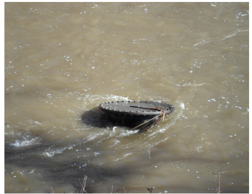
The interceptor of the existing sewer main, dislodged during the storm.
