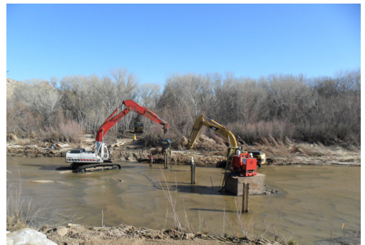
Building a bridge across the Mojave River, to support the bypass piping, was a key component to the solution.
