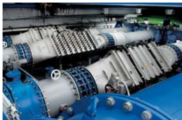
The WEDECO K reactors installed at Wahnachtalsperre (river dam) are certified by the DVGW according to technical standard W294: Biosimetric dose of 400 Joules/m 2 .
