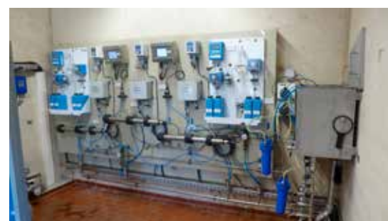
WTW NiCaVis UV 705 IQ NI Multi-parameter online measurement
