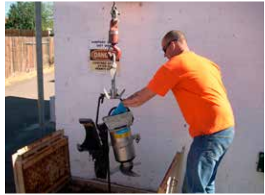
Installation of a Flygt submersible mixer.
