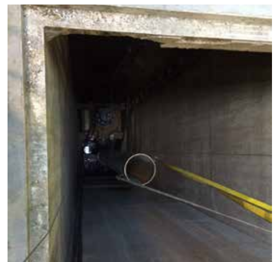
3400 pump and pipe
