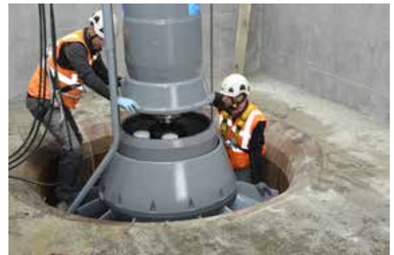
Assembling the generator to the hydraulic unit in one step, without any need of bearing or shaft alignment.
