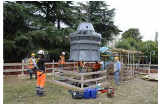
Installation of the hydraulic unit in the power station.
