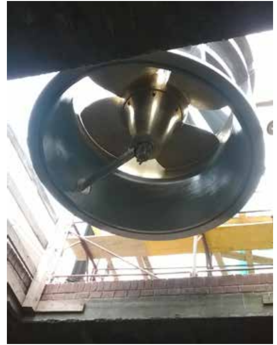
Flygt EI 7650 unit with adjustable bronze blades between 4° ~ 32° inside the outlet cone.
