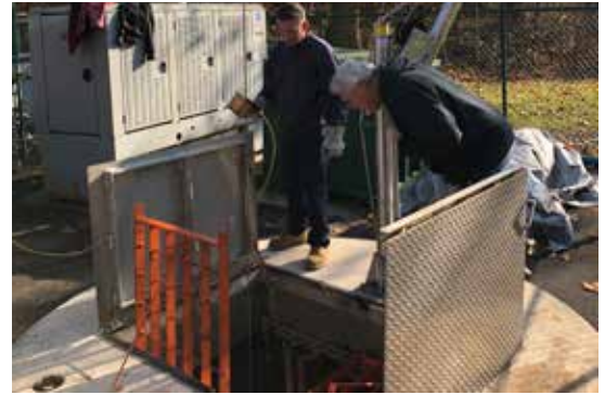
Winch hoisting pump in wetwell for inspection.
