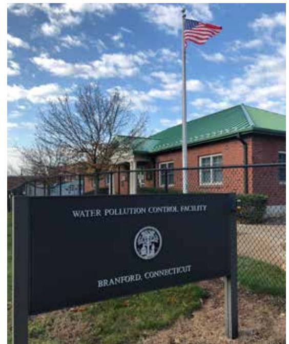
Branford WWTP administrative building.
