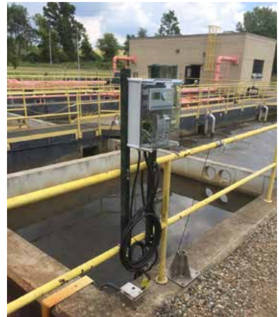
Tank side controls provide easy access to a host of mixer functions.
