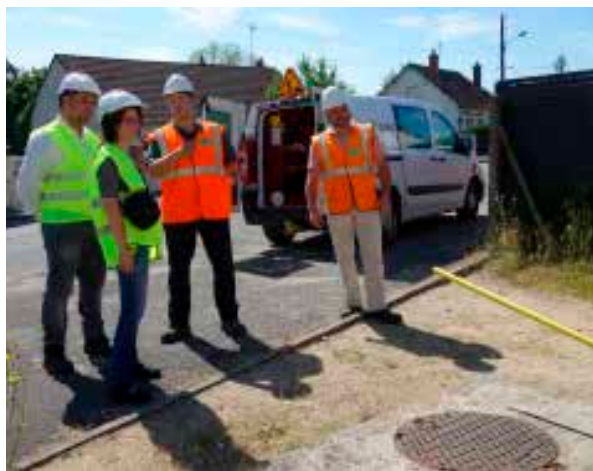
Engineers from Suez and Xylem on site at the Sully-sur-Loire pumping station
