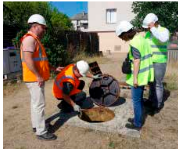
The pumping station is prepared for the installation of Xylem’s Flygt 3069
