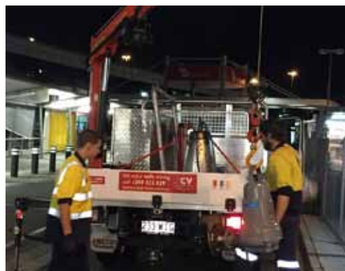
Pump being unloaded with old pump on back of the truck
