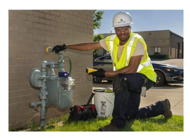
Will Linzy, Nicor Gas meter reader, is installing a FlexNet communication module. The easy installation does not interrupt natural gas service during the few minutes it takes to place the module onto existing natural gas meters.
