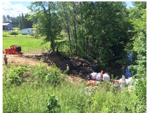
The Godwin power pack was situated 150 feet from the creek, addressing environmental concerns.
