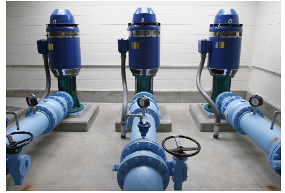
Xylem recommended its Goulds Water Technology vertical turbine pumps as a highly efficient, reliable, and easy-to-operate solution that could be configured for new pit depths.
