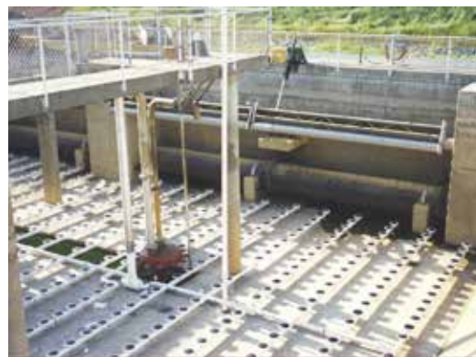
The Sanitaire fine bubble membrane grid aeration system
