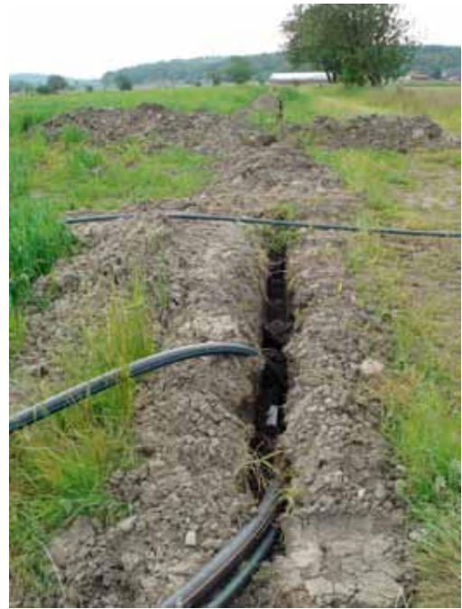
Trench for the PSS sewer collection network.
