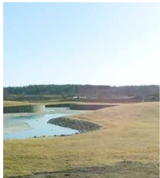
Myra Golf Course, adapted PSS installation with minimal impact.
