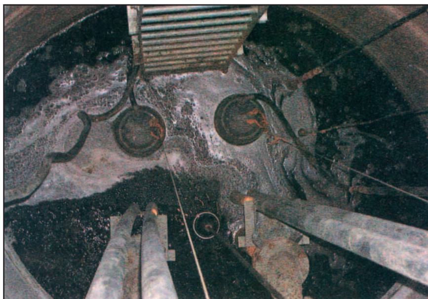
View into the wet well showing the larger, replacement ITT Flygt pumps now in operation at the duplex lift stations.
