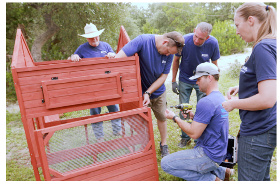
Xylem employees build a new chicken coop to accommodate the family’s chickens.
