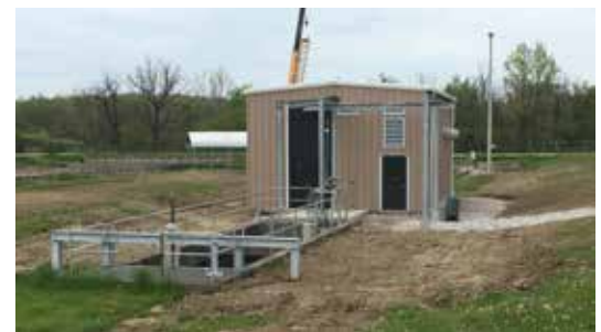
Retrofitting the outdated Trojan 4000 UV system to the Wedeco Duron UV system is easy to perform in the existing infrastructure.
