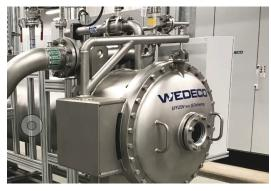
The Xylem-designed AOP system consists of two Wedeco PDOevo 900 ozone AOP systems, each producing 1,000 pounds of ozone per day.
