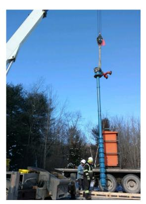
Xylem's field team installed high-lift Goulds Water Technology vertical in-line turbine pump down into the well shaft with a connected Godwin variable frequency drive and MJK flowmeters provided greater visibility.
