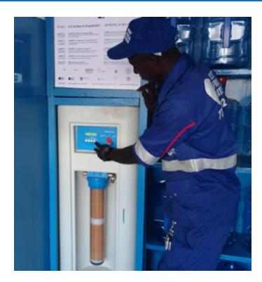
Swiss Fresh Water's BW Delta Treatment system is capable of delivering up to 4,000 liters (1,057 gallons) of purified drinking water per day.
