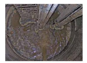
As well as a heavy flow of wastewater, the station also takes in storm water, often including large quantities of solids, which led to frequent clogging issues.
