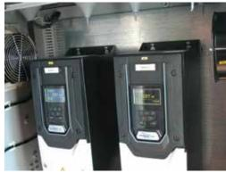
Flygt SmartRun intelligent pump controllers reduce system clogging with automatic sump cleaning and pipe flushing functions.
