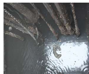
Fig 8: Wet pit surface after
